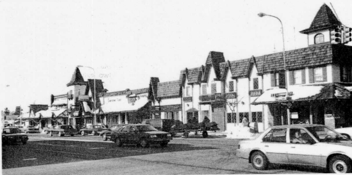
Today, the 300 block shows a face that has been changed and updated over 25 years.
