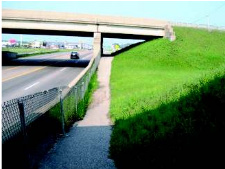
4. View looking west along the north side of West M-32 from the west side of the northbound I-75 bridge.
