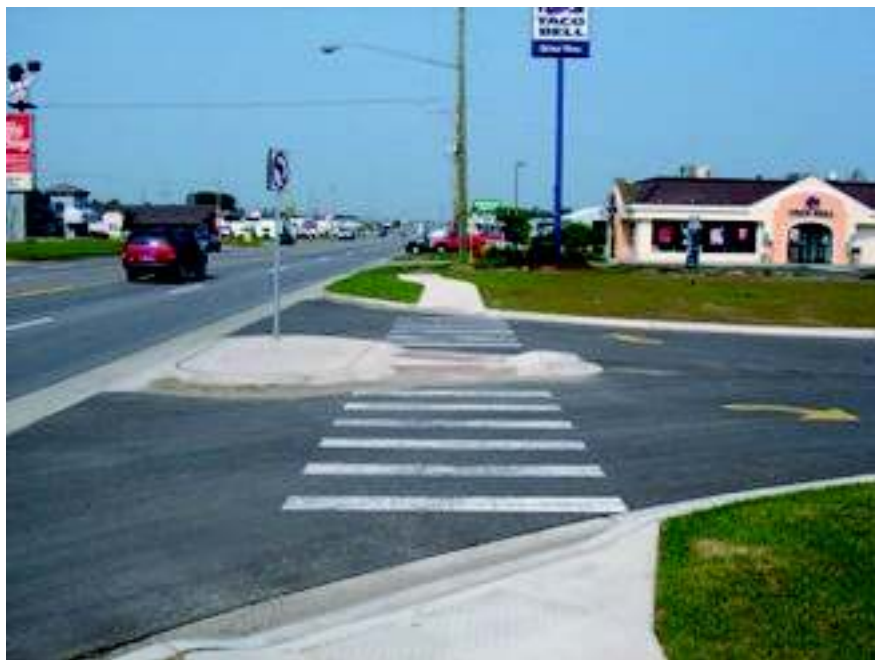
14. View looking west along the north side of West M-32 ROW from approximately 200' west of the Meecher Road intersection.
