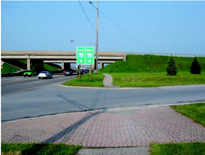
1. View looking west along north side of M-32 at the Northbound I-75 entrance ramp and the start of the West M-32 Streetscape segment.
