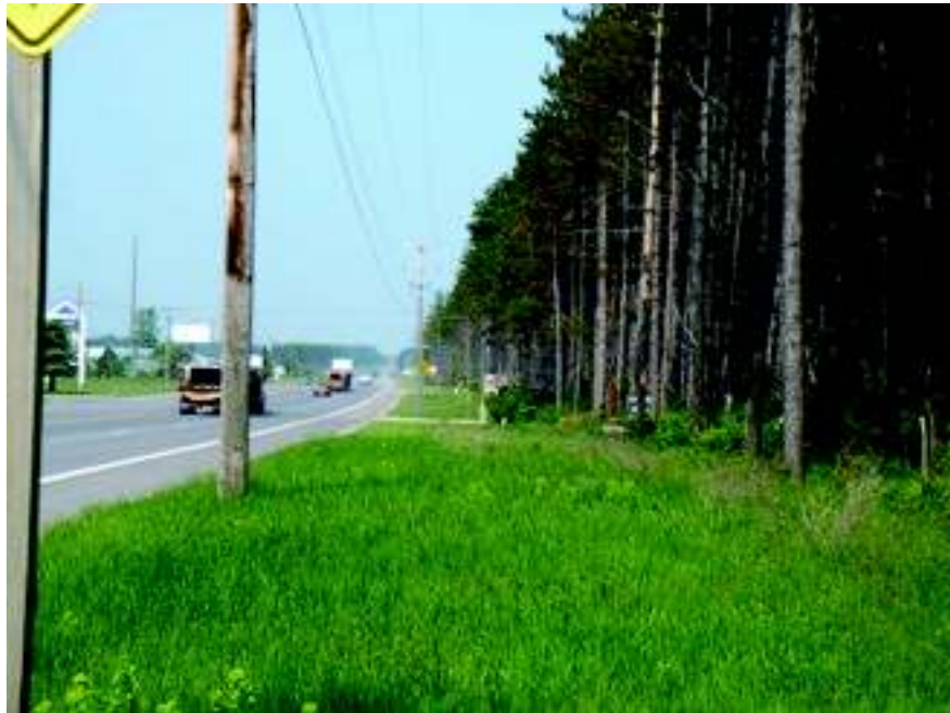
4. View looking west along the north side of M-32 and power line ROW from approximately 400' west of the Murner Road intersection.
