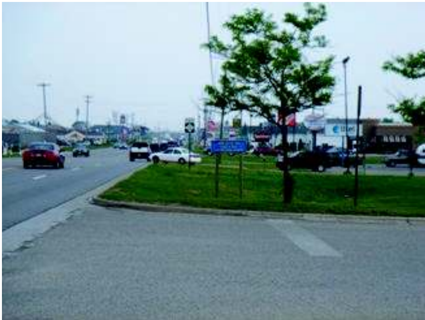
24. View looking east along the south side of West M-32 ROW from approximately 550' east of the Murner Road intersection.
