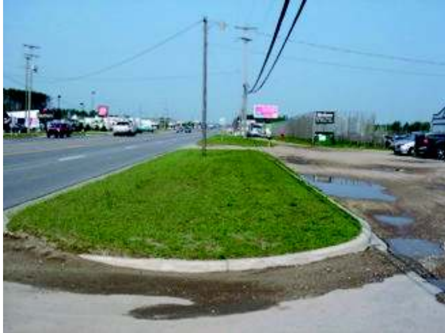
17. View looking west along the north side of West M-32 ROW from approximately 800' west of the Meecher Road intersection.
