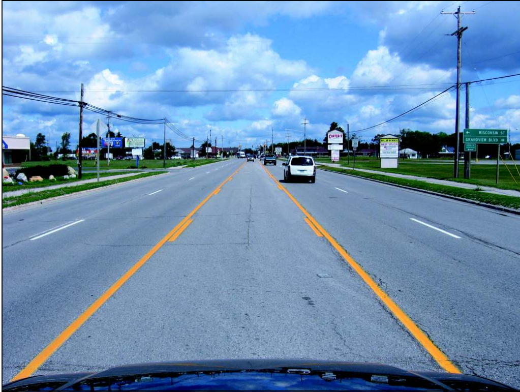
23. View looking north along South Otsego Avenue from approximately 500' north of the Commerce Blvd. intersection.
