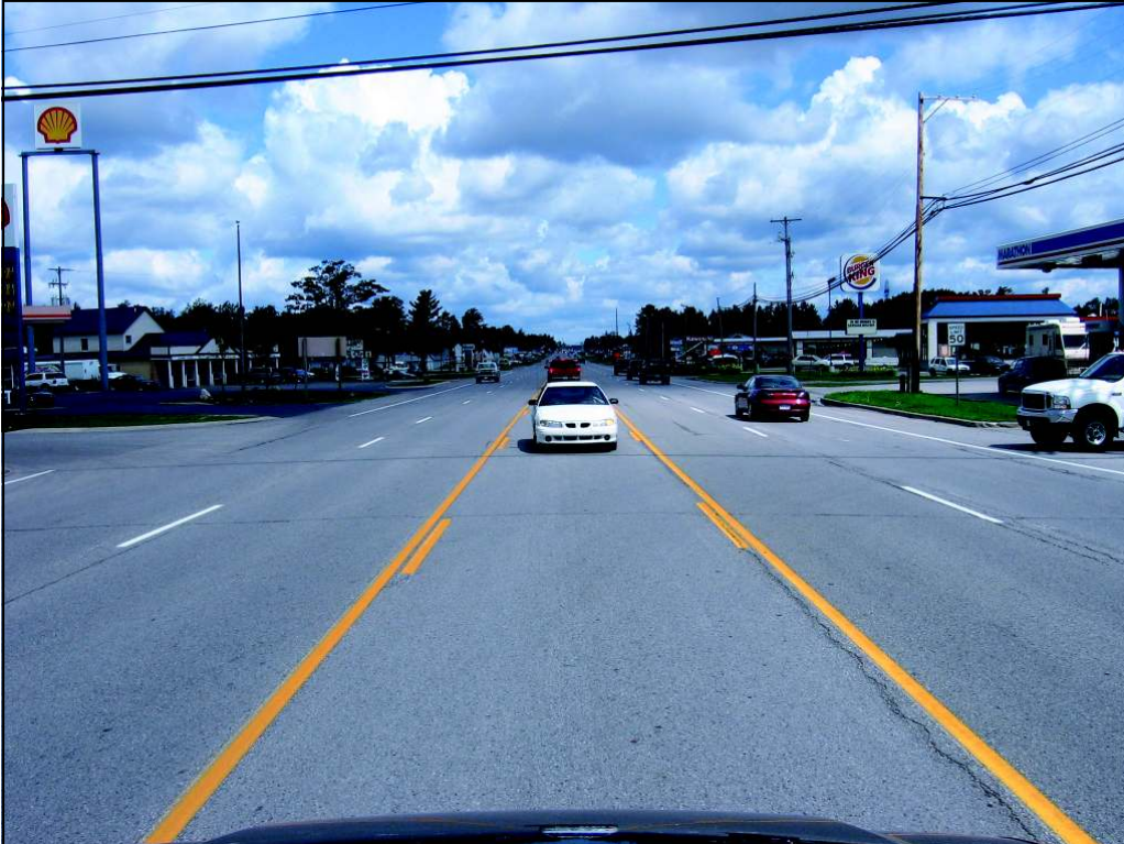
2. View looking north along South Otsego Avenue from the intersection with Driftwood Lane.
