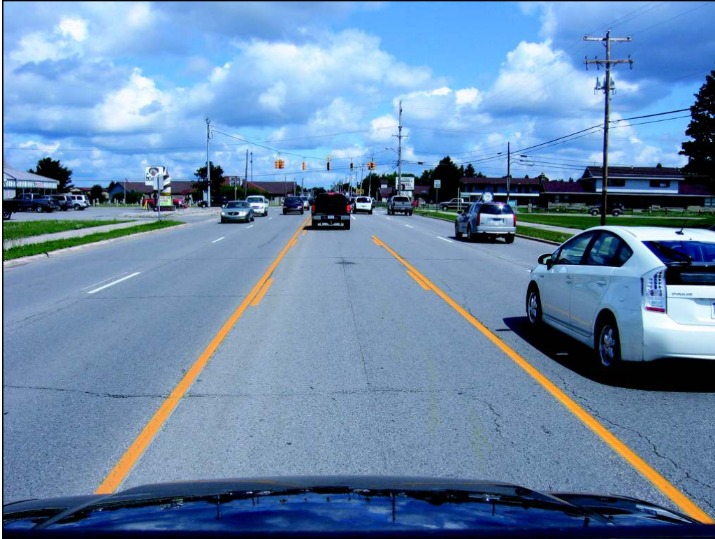
25. View looking north along South Otsego Avenue from approximately 300' south of the South Wisconsin/Grandview intersection.
