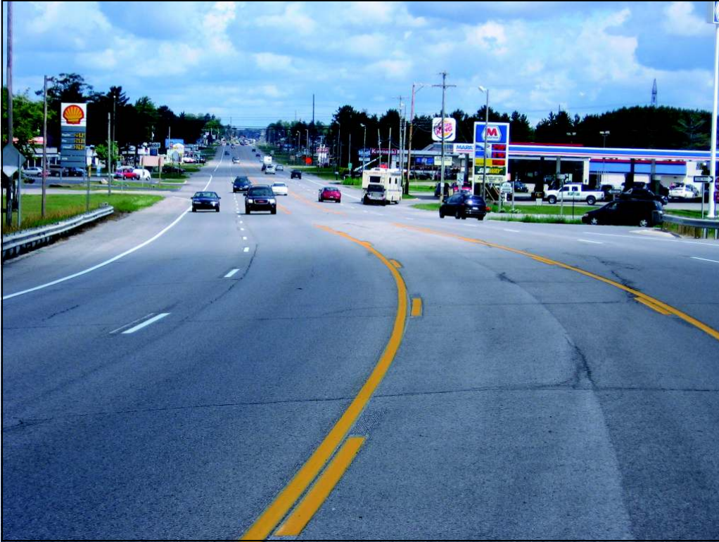
1. View looking North along South Otsego Avenue from the north end of the overpass at I-75.
