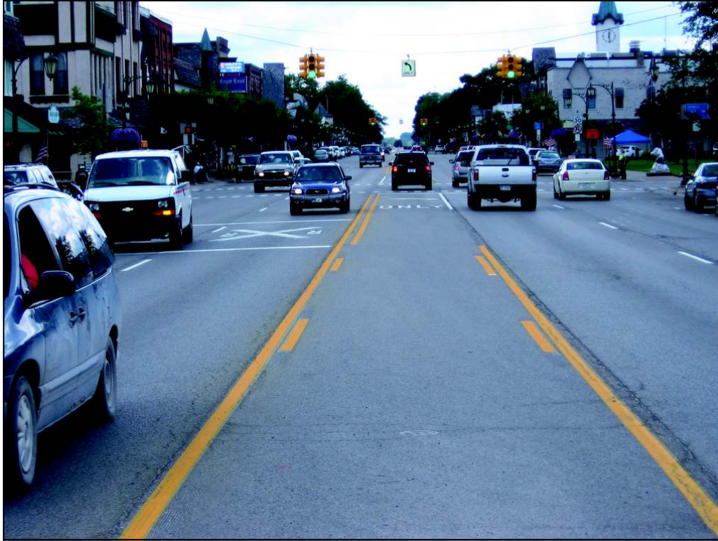
View looking east on Main Street from just west of the Otsego Avenue intersection
