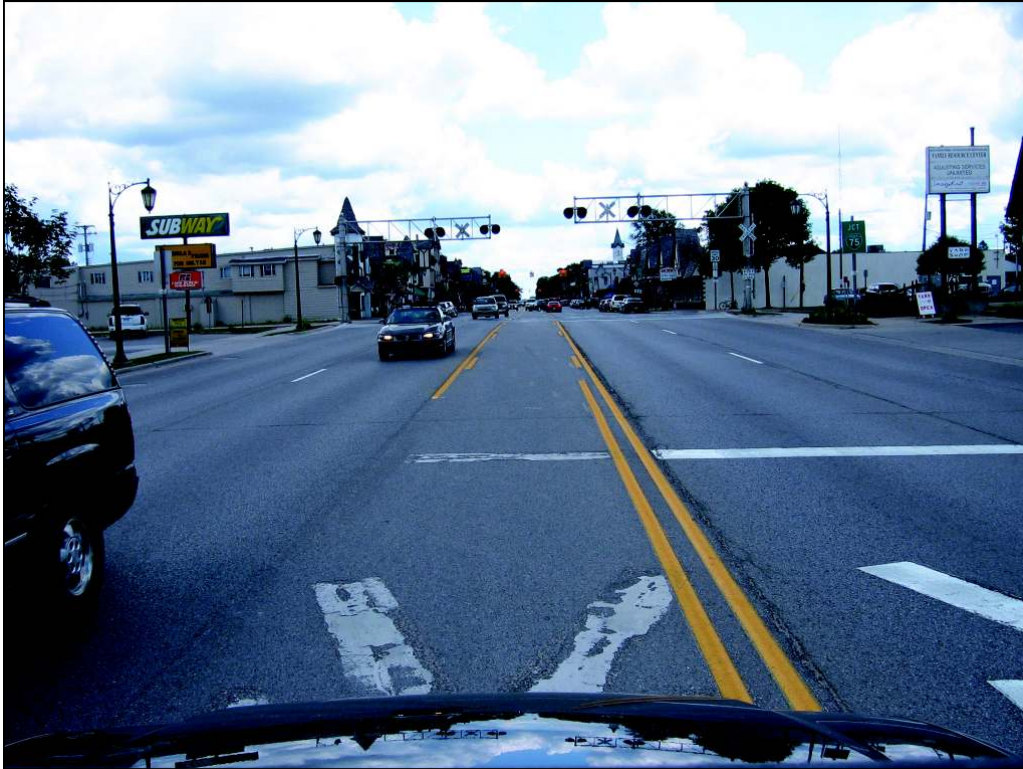
View looking east on Main Street towards rail road crossing and start of project area. The first project segment is located at the railroad crossing (snowmobile trail crossing safety improvements)
