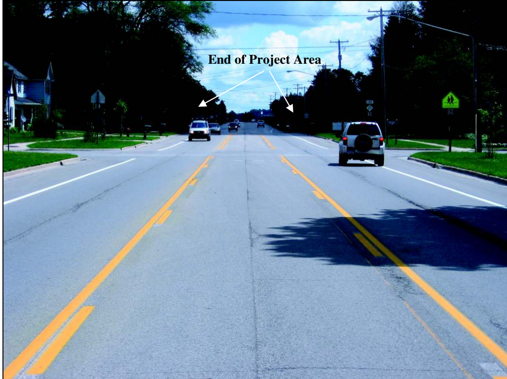
View looking east on Main Street from just west of the Maple Avenue intersection. End of third project segment project area is noted on photo.
