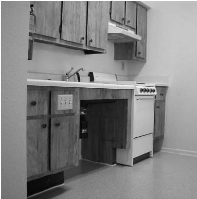
This kitchen area includes a roll under sink area, lever handle faucet, and a stove/oven unit with controls up front
